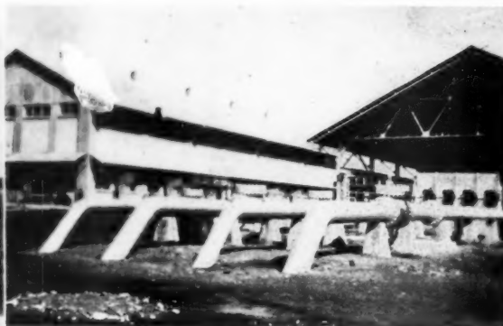
Start of present 12 and 16-in. I.P.C. pipe-line system at Kirkuk Station K-1.
